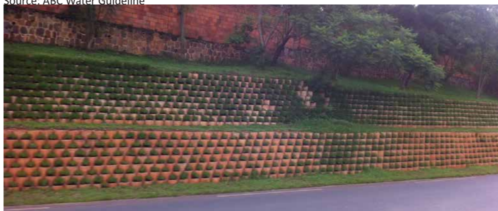
Fig.3.43 Green Retaining Wall
