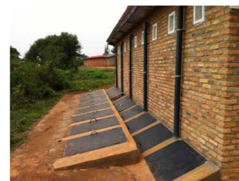
Fig.3.33 Compartment to Separate Human Waste in EcoSan
