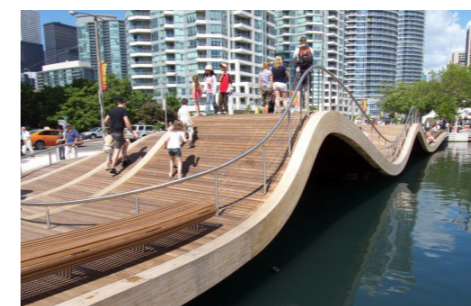
Urban Recreational facilities
